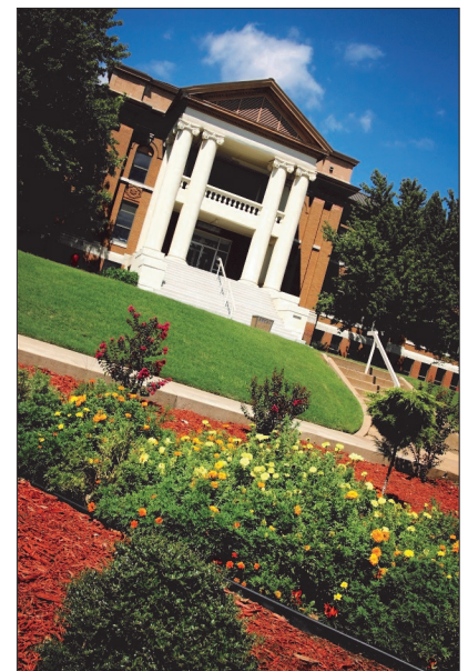
SWOSU's "Old Science Building" was built in 1909 and is on the National Register of Historic Places
